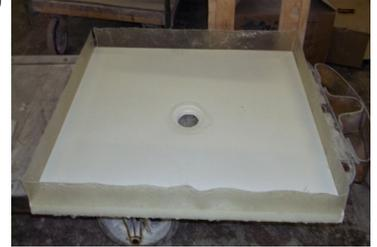
**Step 2.** Set the shower base in place. The base should be set directly against the wall studs. After the base has been set, use a water-resistant wall covering such as green board to establish the wall face. The wall covering will meet the shower floor therefore concealing the fiberglass edging on all sides but the door opening. The fourth exposed side is concealed through construction of threshold. This threshold also creates the horizontal surface on which to mount the door.
